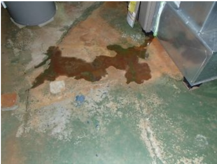
condensate leaking
