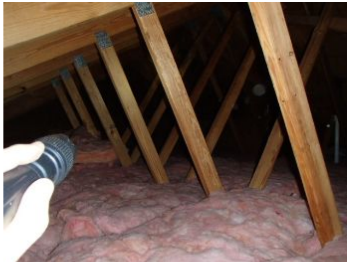
garage attic area
