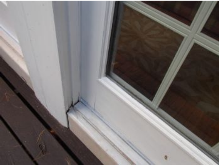
water damage to doors
