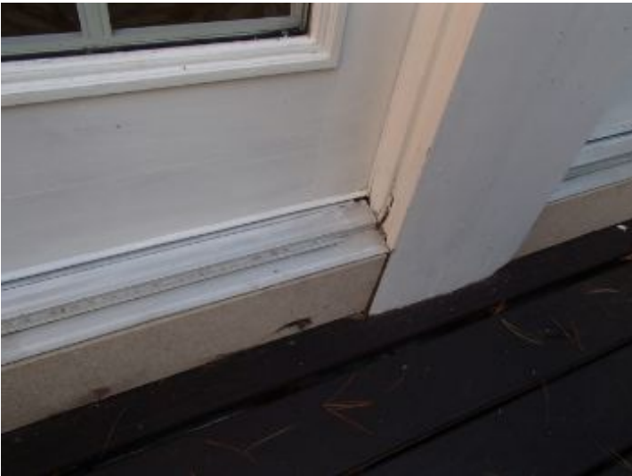
water damage to doors
